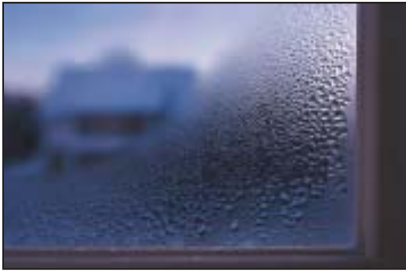
Condensation on the inside of a windowpane.
